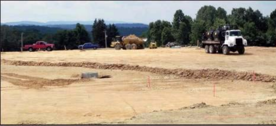
Michelle Wolford/The Dominion Post Workers do site preparation behind Tunnelton-Denver School for a new South area school.
